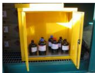
Inside a safety cabinet for flammable substances
