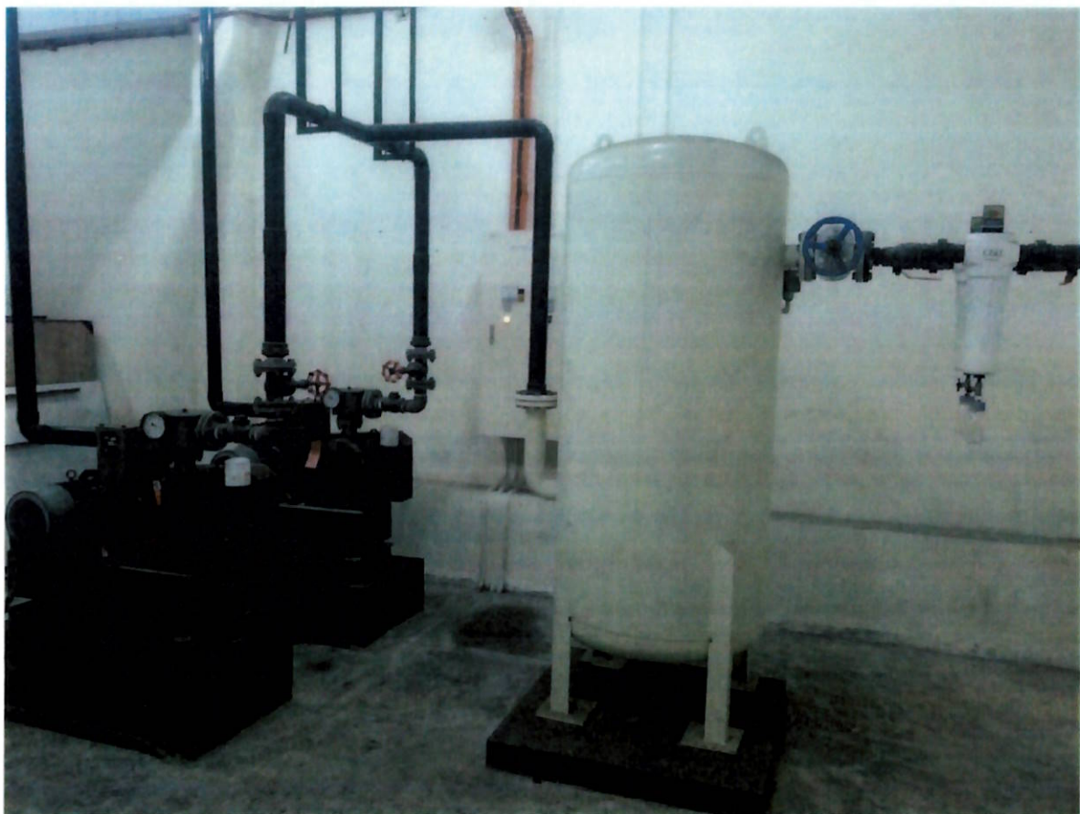
Figure 1. Vacuum System at PMMPMHAMB Hospital.
