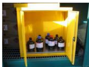
Inside a safety cabinet for flammable substances
